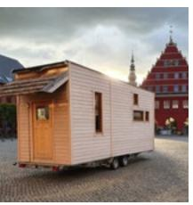
**Properties** The Tiny House was built using as many paludiculture materials as possible: cattail for insulation, reed and wet grass panels for interior finishing, and alder wood for the supporting structure. It is transportable, fully equipped, and suitable for repeated use. It demonstrates climate-positive construction in a practical and tangible way, at a 1:1 scale.
