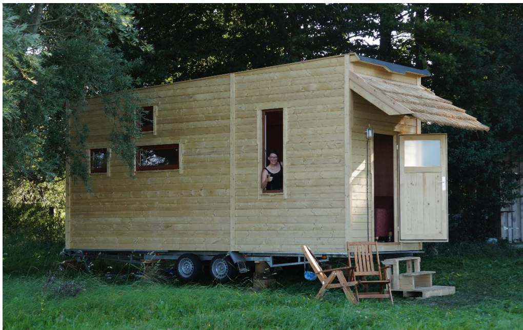
Fig. 1. Tiny house made with building materials from paludiculture plants (Photo: A. Nordt).
